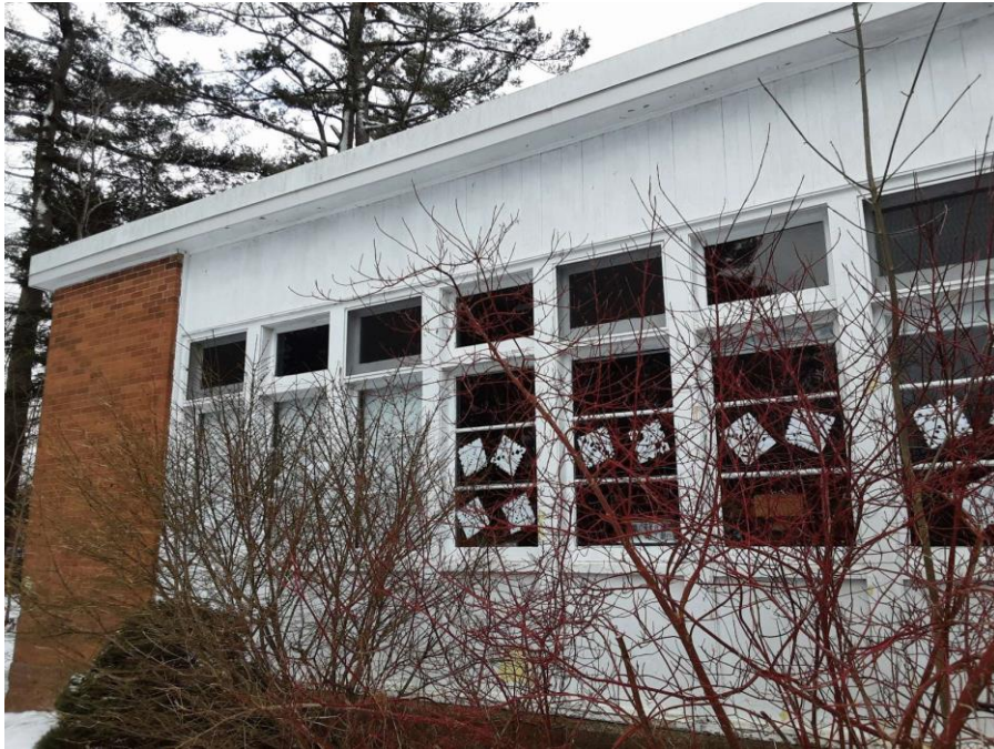
L0002, White paint on wood siding, Exterior (Location #: 1)
