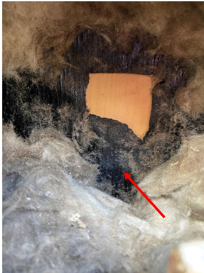
None-Asbestos Tar Paper (S0009A-C) and fiberglass insulation inside exterior wall, Exterior (Location #: 1)
