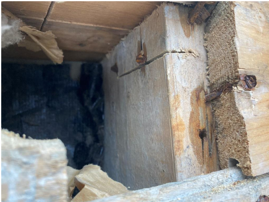
Intrusive investigation to exterior wall , Exterior (Location #: 1)
