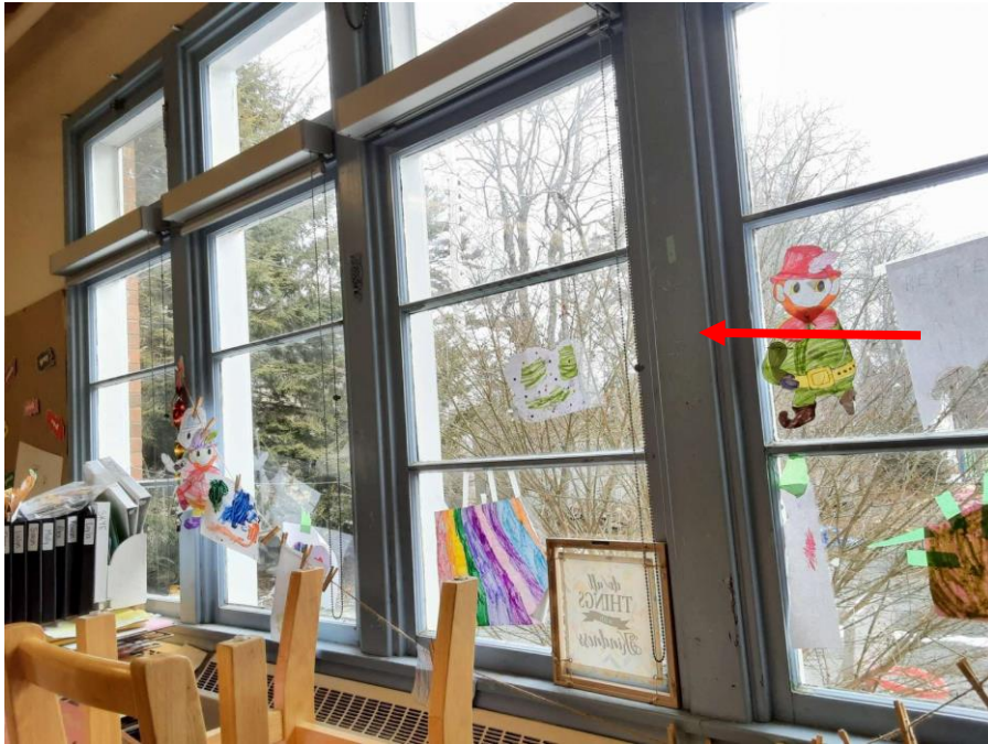
L0004, Light blue paint on wood window frames, Classroom 6 (Location #: 2)
