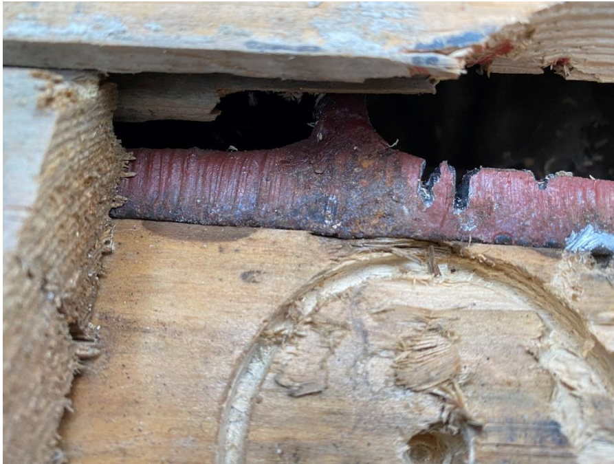
Intrusive investigation to exterior wall, Exterior (Location #: 1)
